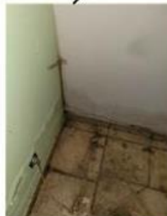
Trace de termites souterrains (cordonnets)
